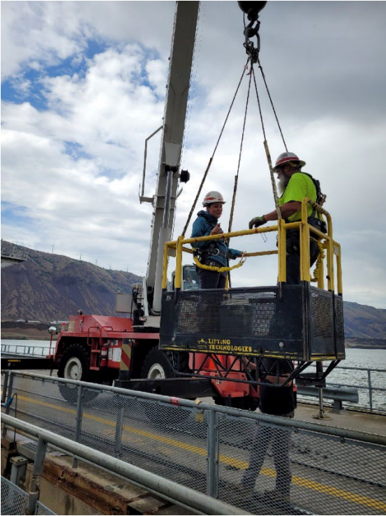
Fish recovery on bulkhead.
